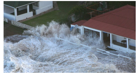
Inappropriately placed engineering infrastructure can make coastal homes more vulnerable to sea surges instead of protecting them. Eden District, South Africa.
